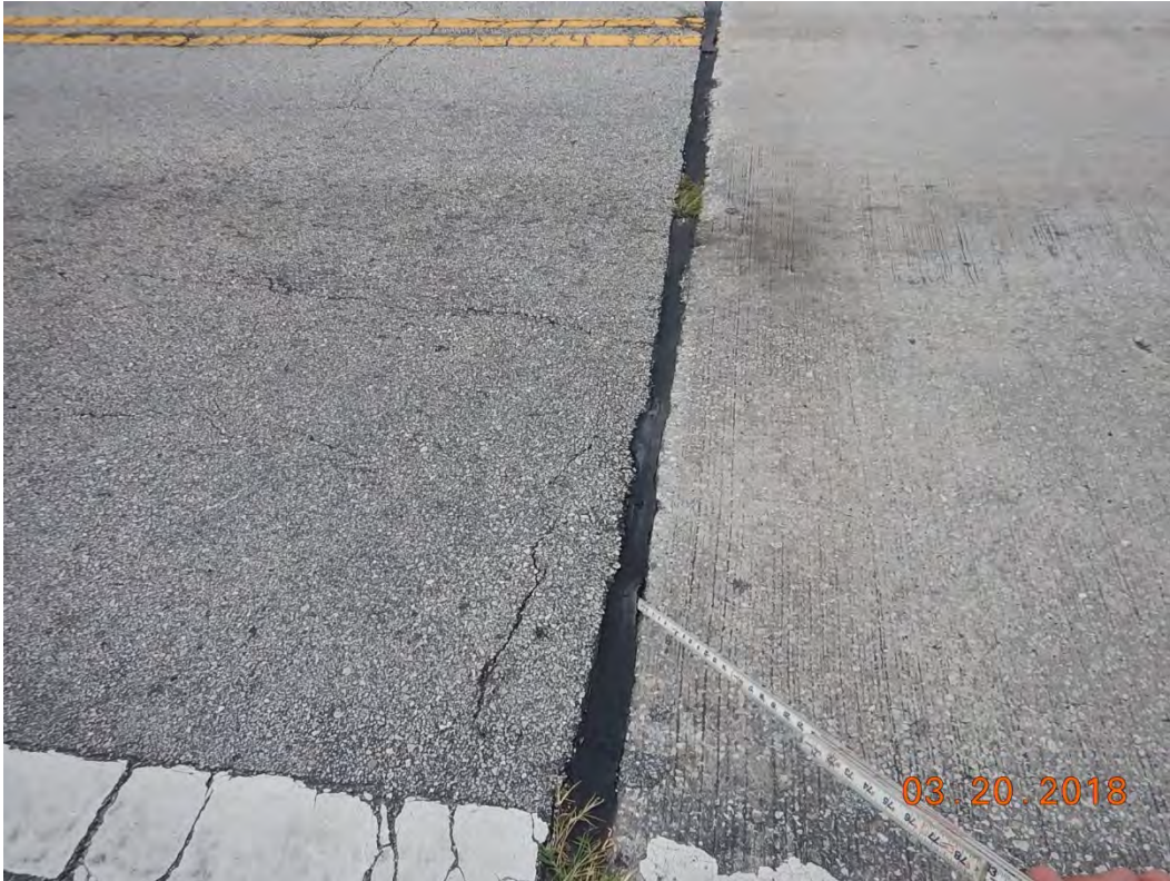
Photo 3: Element 301: Showing typical adhesion failure of expansion joint sealant.
