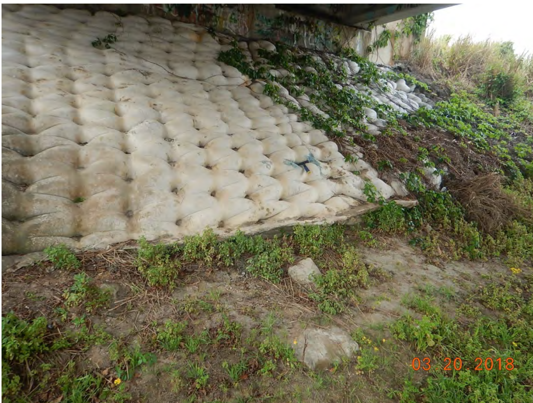
Photo 6: Element 8396: Showing vegetation growth at north slope protection.
