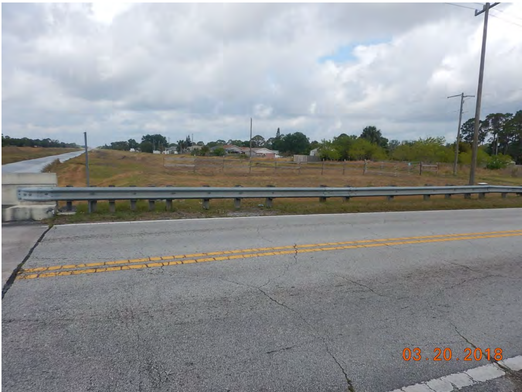
Photo 8: Inspection Notes: Showing broken and missing guardrail mounted reflectors.
