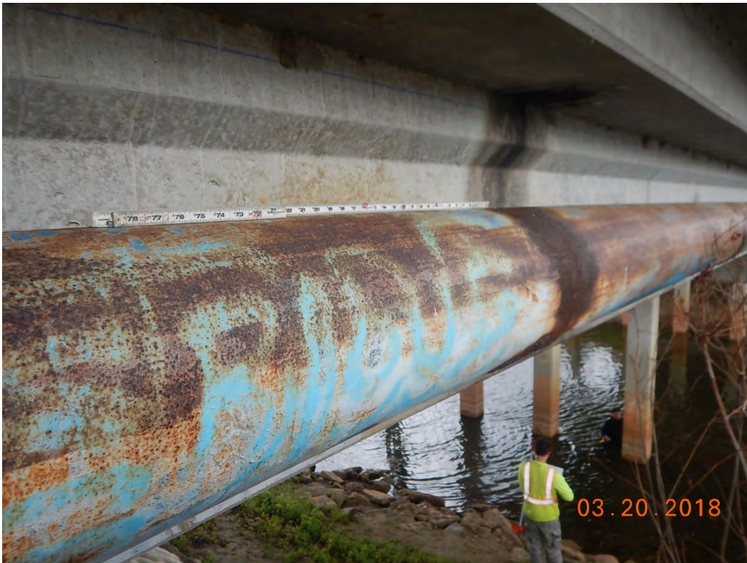
Photo 2: Element 8098: Showing heavy corrosion and leaking utility pipe on right side of the structure.
